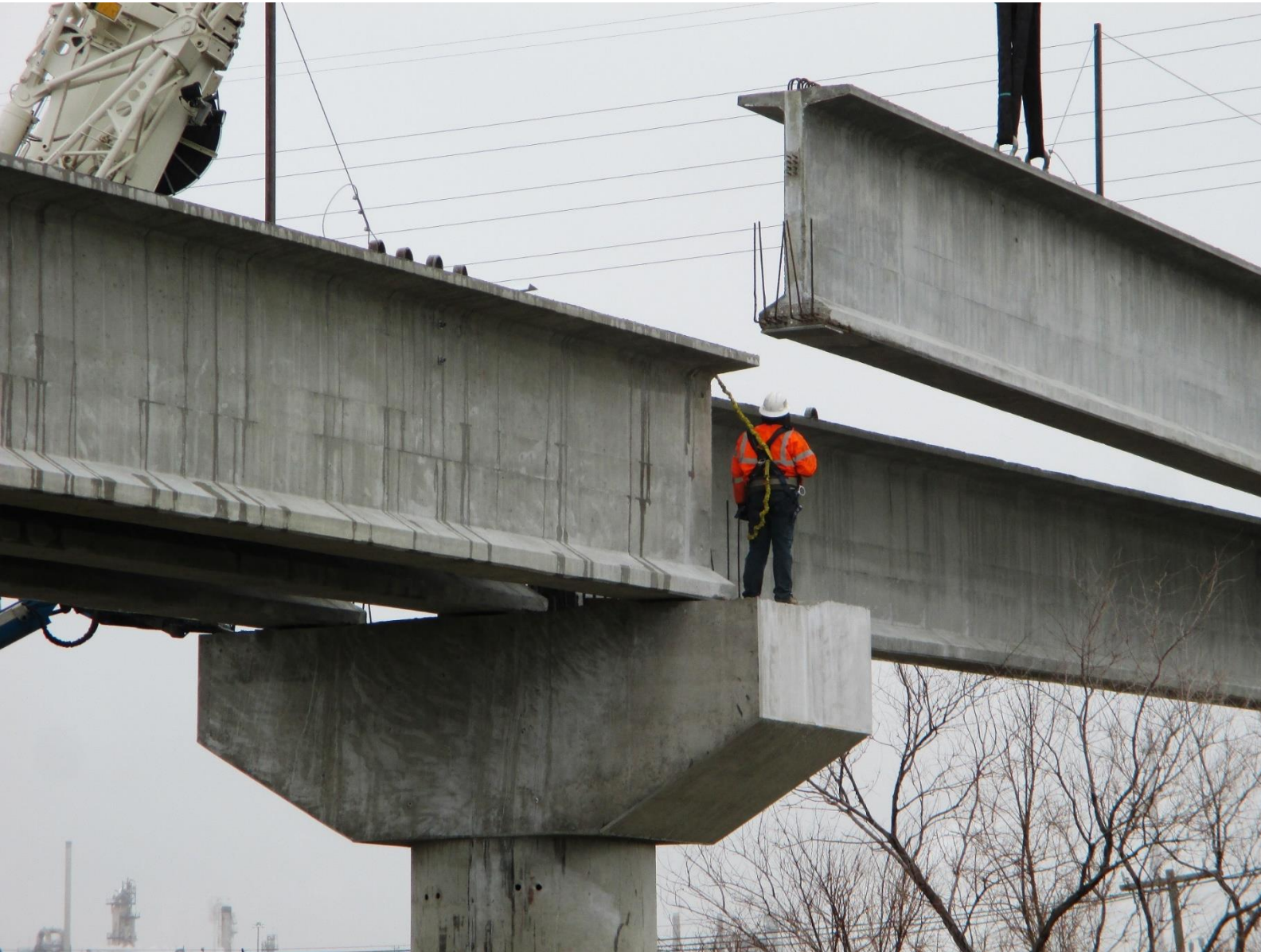
Photo Courtesy Regional Transportation District.
